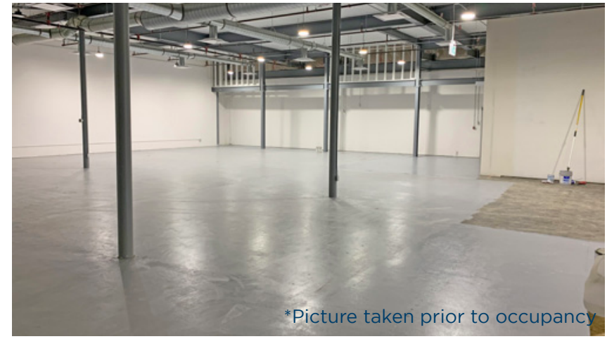
*Picture taken prior to occupancy
