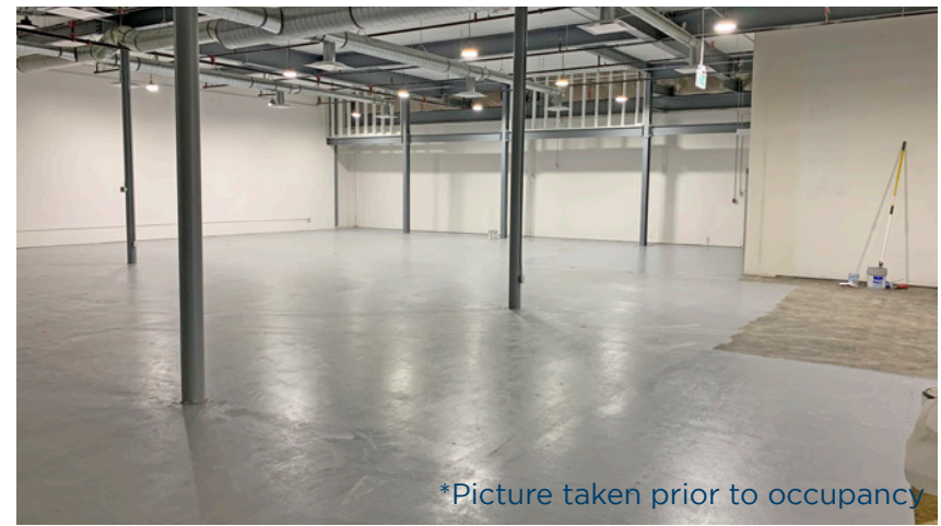
*Picture taken prior to occupancy
