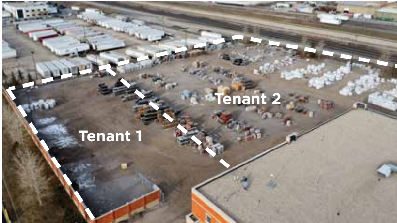
Yard area, unpaved (Tenant 1) // NW side of building
