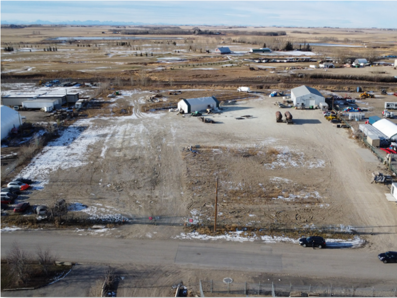
Features: // Compacted and fenced site
